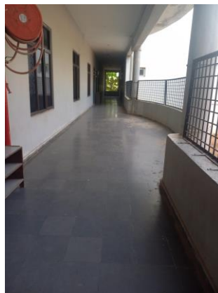
Corridors with daylight
