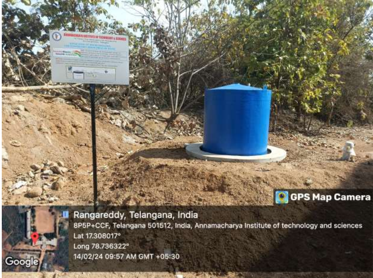
Bio Gas Plant at AITH
