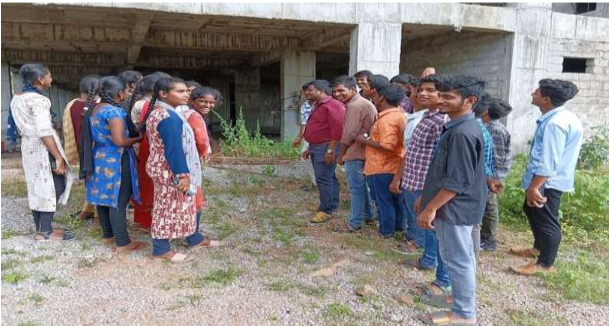
Field visit Construction Site TS Govt. Double Bed Rooms at Piglipur Village
