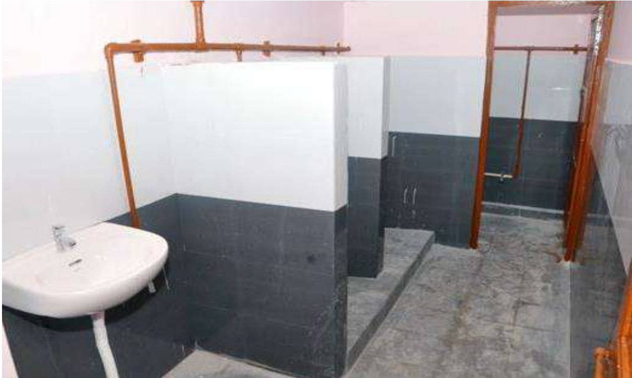
Wash Rooms for Disabled.
