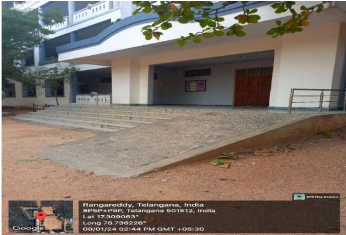
Pedestrian Friendly Pathway Ramp at Block - B AITH
